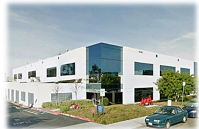
DNA Production Facility (San Diego)
